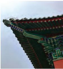
Longfu Temple roof detail uses sunmao construction methods
